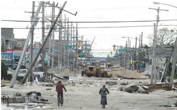
Root cause analysis conducted after the storm underscored the critical role that poles play in our power infrastructure. When all the statistics were in, customer-affecting outages in the distribution network were found to be caused by damage to an eye-popping 18,617 poles and their associated aerial lines and transformers<sup>4</sup>.
