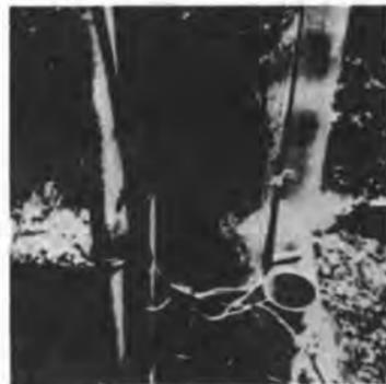
C — Showing spare conduit right foreground-uncapped. Half round metal conduit covering live conductors rear of spare.
